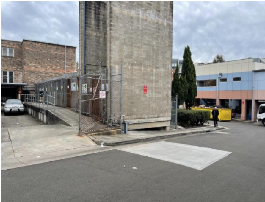
Figure 2 - Existing filling point hard stand
